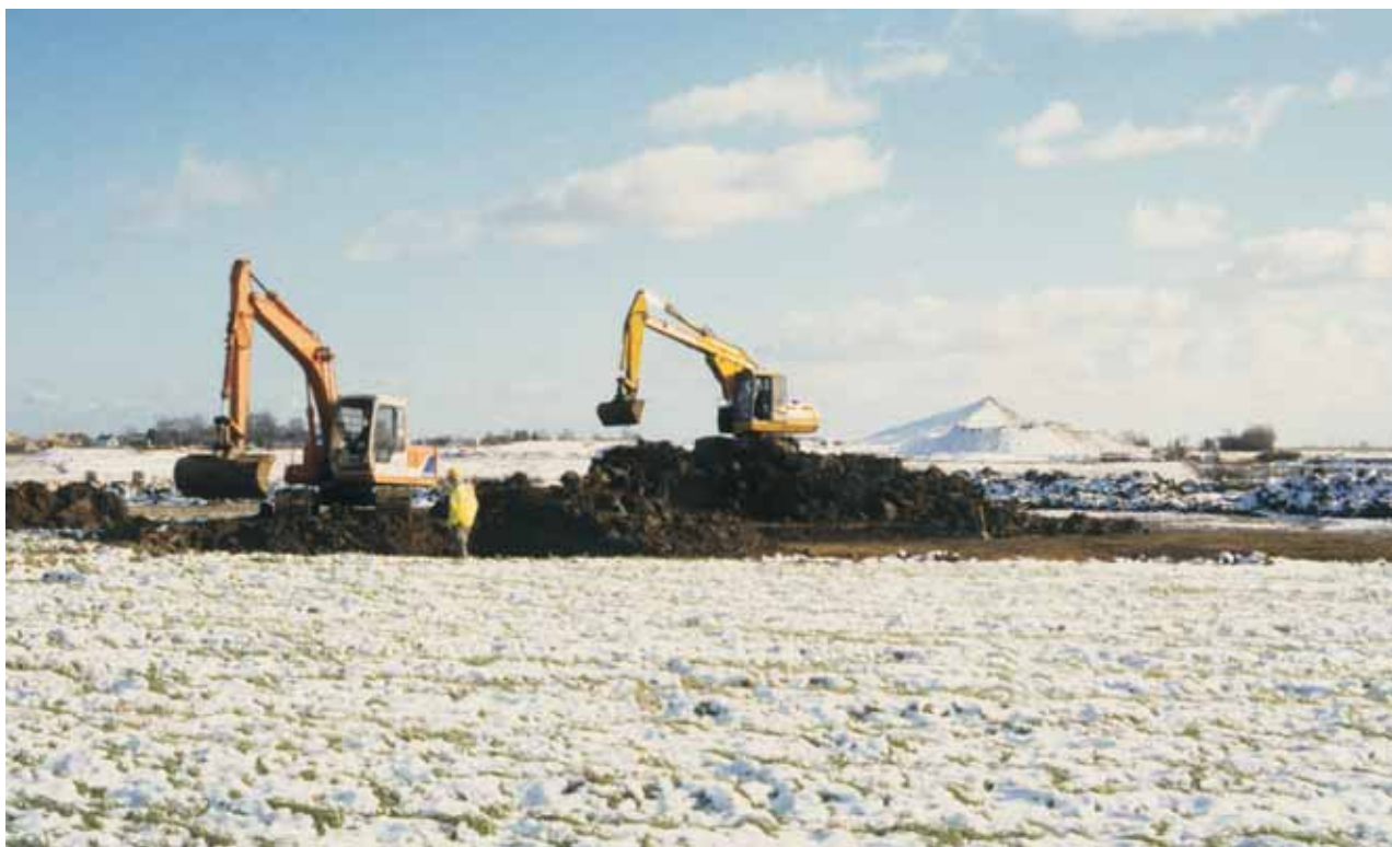
Plate 3 Topsoil stripping at Lower Cambourne in winter
