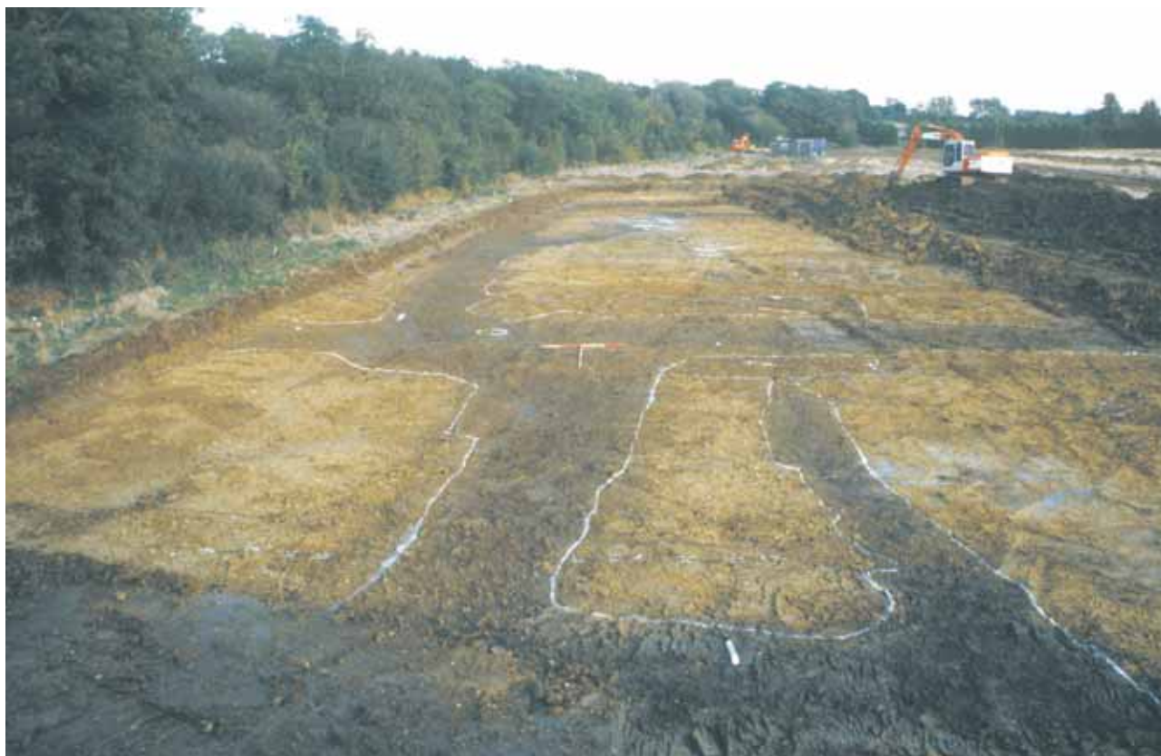
Plate 16. Knapwell Plantation: machining in progress, revealing enclosure ditches
