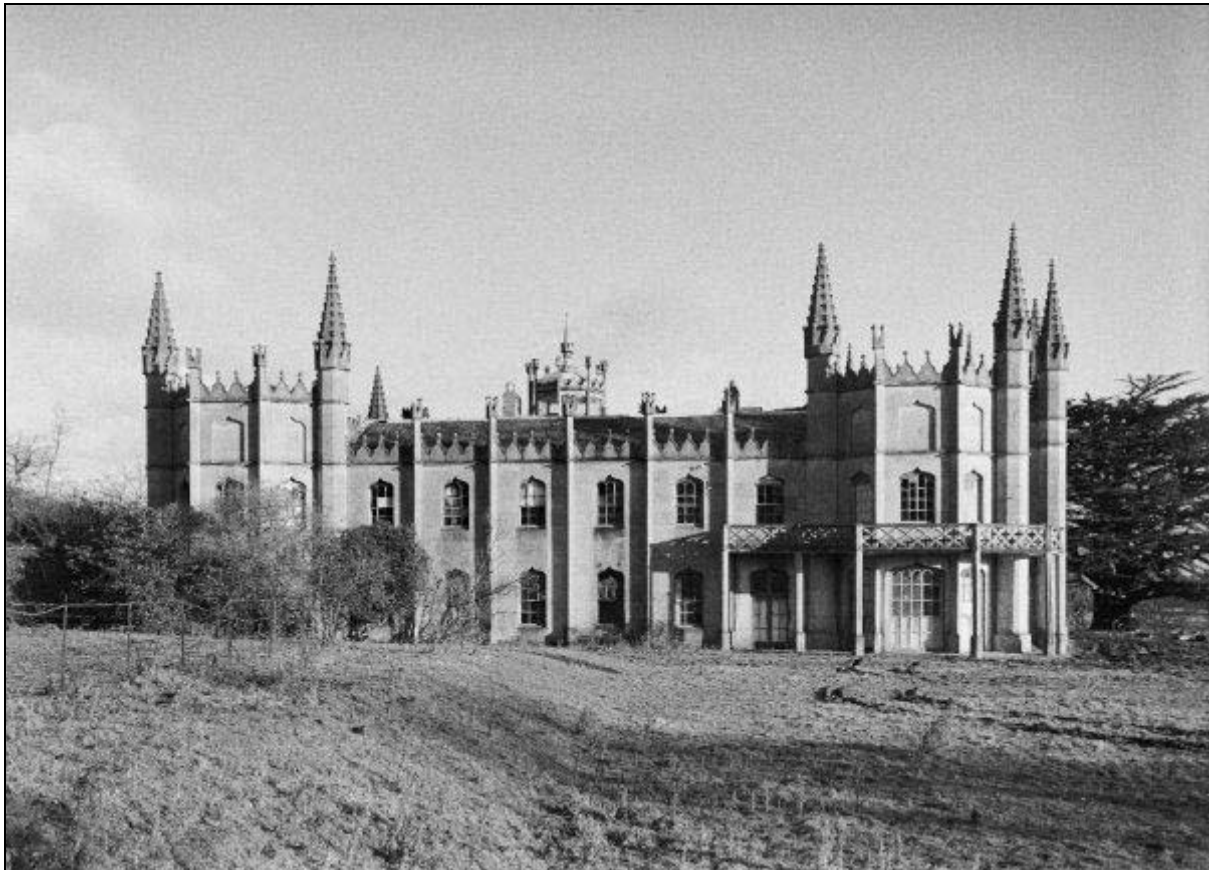
Figure 6. Photograph of Garth Hall in 1947: The hall was demolished in 1950-52. It was built at great expense in 1809 for Reverend Richard Mytton, chaplain to the Governor General of India, in a bold mixture of gothic and ecclesiastical styles by the well known garden designer and writer, John Claudius Loudon. (© Crown Copyright: RCAHMW DI2008_0839).
